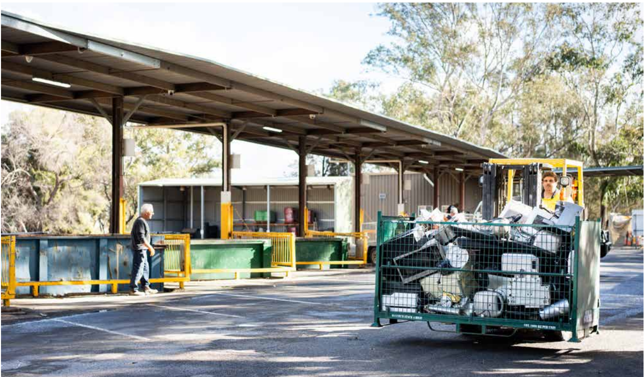
Resource & Recovery Waste Transfer Station
