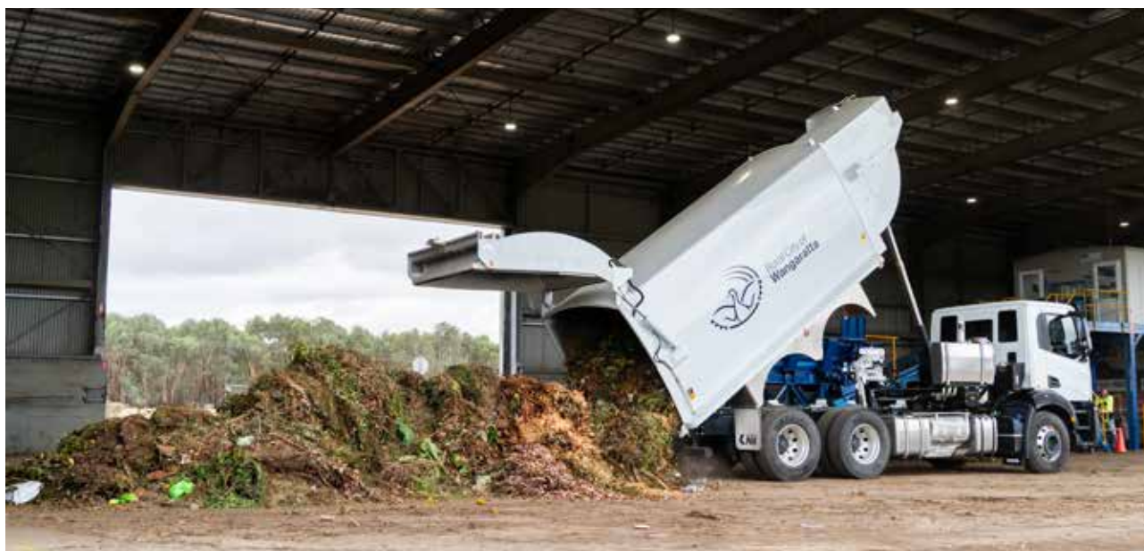
Wangaratta Organics Processing Facility
